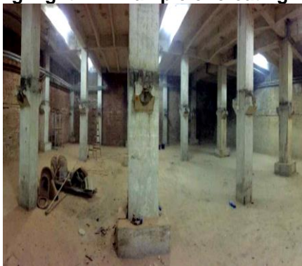
Before (550 m 2 unrentable space)
